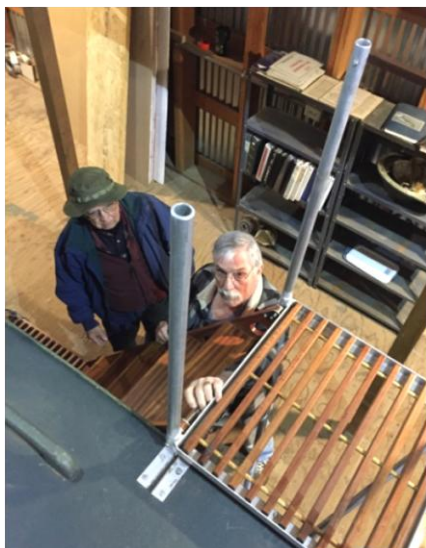
Installing The Boarding Ladder
