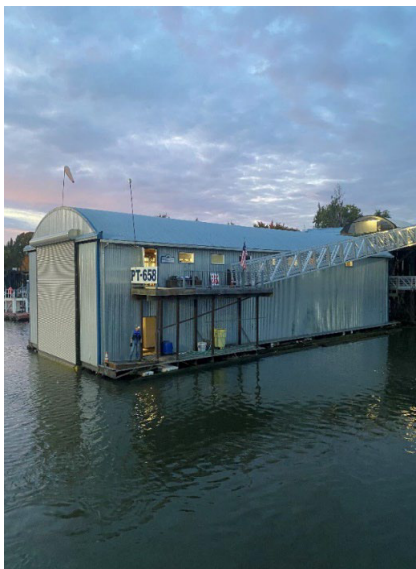
Our boathouse with a newly installed door
