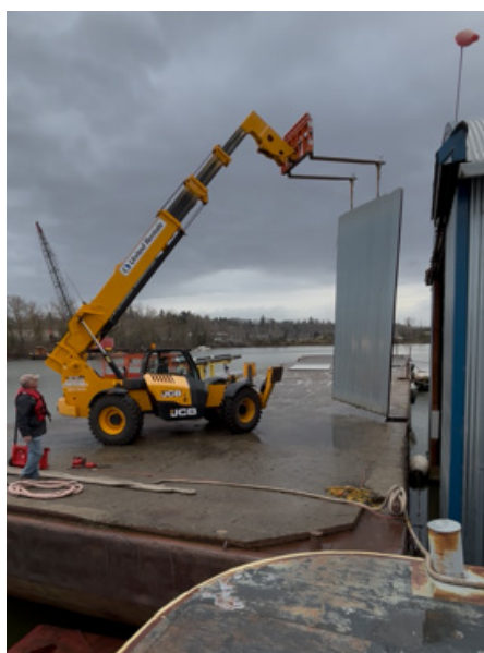
Removing the old door.
