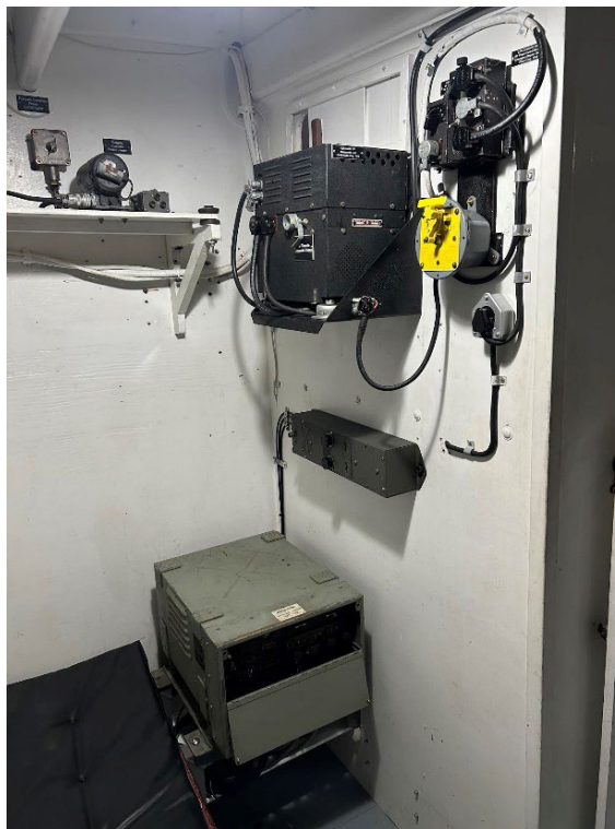
BN unit fully installed on PT 658
