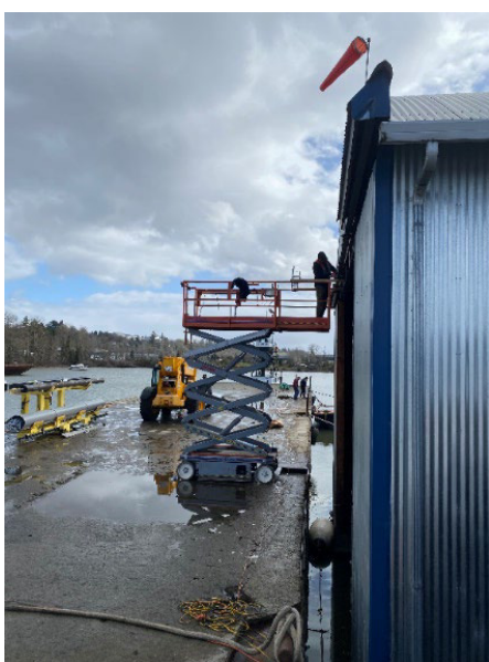
Tom Voight Hanging the New Door
