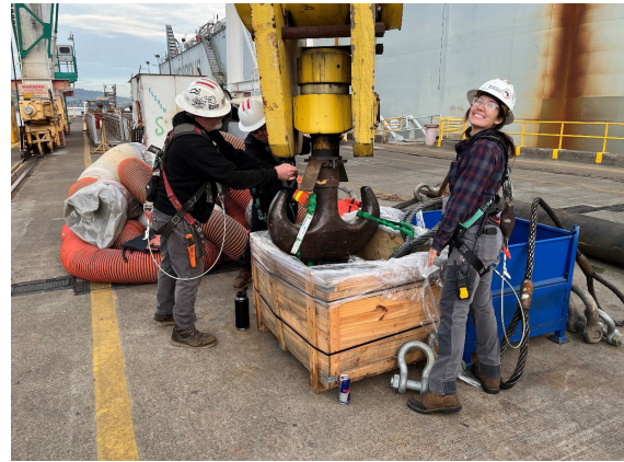
Vigor crew preparing rigging to lift the 658
